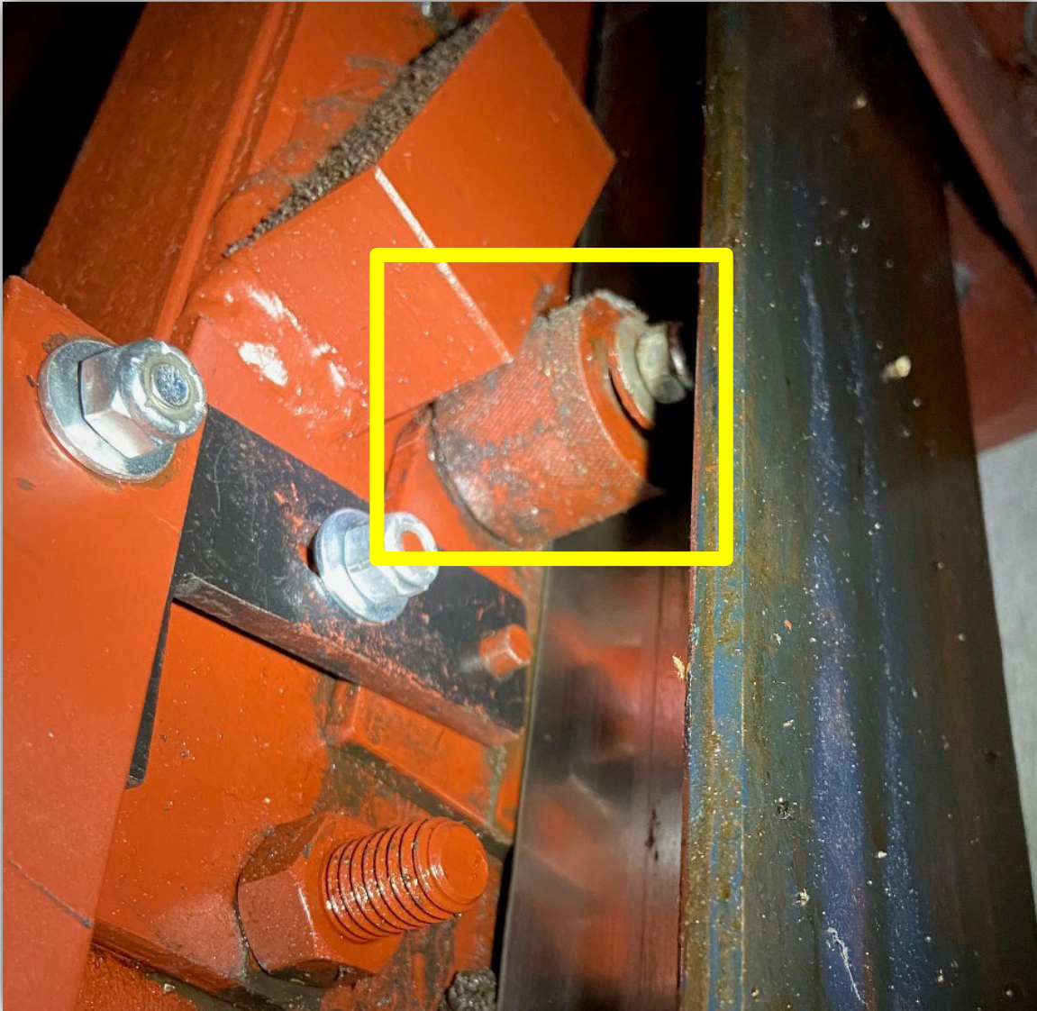
Photo 5 – Safety roller with paint
