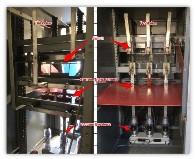
Photo 11 - Unit #6 'prior' to incident with front side and backside views.
