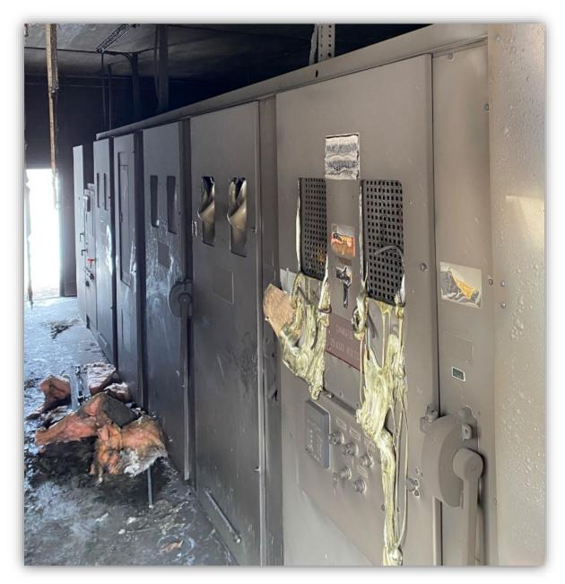
Photo 9 - Front view of 25kV switchgear, module closest is #6- chip mill where majority of damage occurred in the back of the unit, next unit is #5 where initial stress cone fault occurred in the back of the unit.
