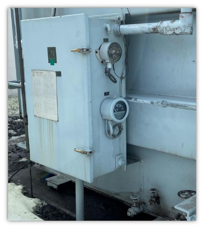
Photo 5 - Transformer control cabinet with gauges.
