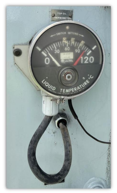
Photo 6 – Transformer oil temperature gauge with red indicator showing oil temperature reached nearing 110 degrees Celsius.
