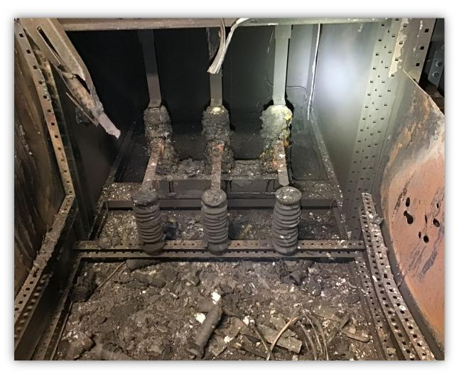
Photo 12 – Unit #6 after incident with back cover removed. Cables through floor no longer exist and are burnt off at floor level.
