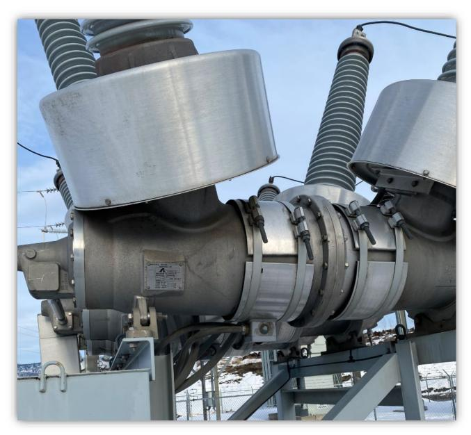
Photo 2 - Close up view of SF-6 breaker equipment with electric heating bands.
