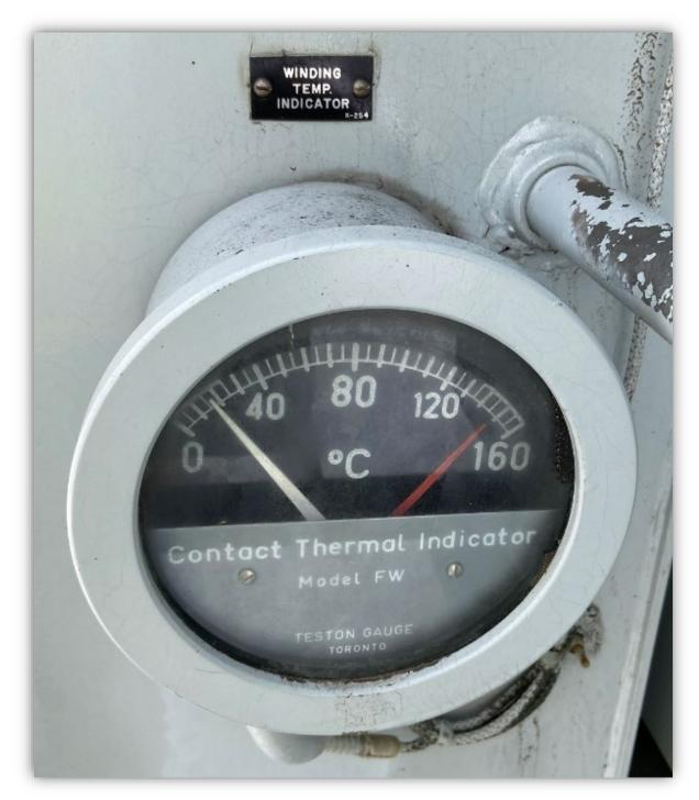
Photo 7 - Transformer winding temperature gauge with red indicator showing winding temperature reached 145+ degrees Celsius.
