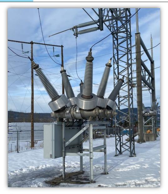
Photo 1 - 138 kV SF-6 main overcurrent breaker, first and only overcurrent protection prior to the switchgear disconnects, Breaker was in 'lock out mode' due to insufficient gas pressure.
