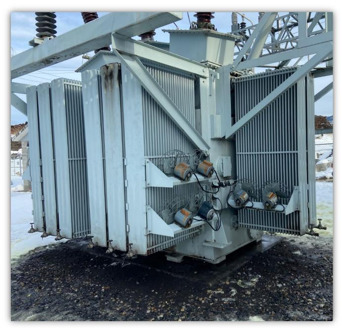
Photo 4 - 138-25 kV transformer showing oil spillage on ground.
