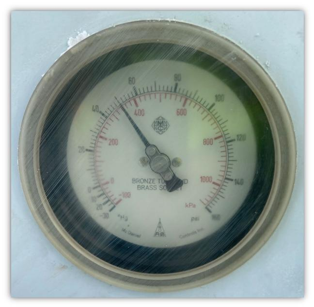
Photo 3 - SF-6 breaker gas pressure at time of assessment at 50 psi. Low Pressure alarm is triggered at 76 psi and breaker lock-out mode is 72 psi preventing breaker from operating.
