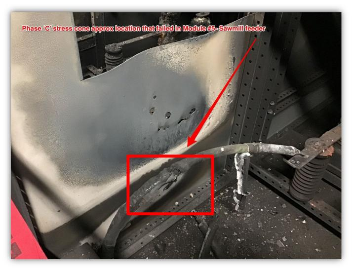
Photo 13 - Module #5 with cable laying in approximate location of operation, the cable has a noted fault on the stress cone.
