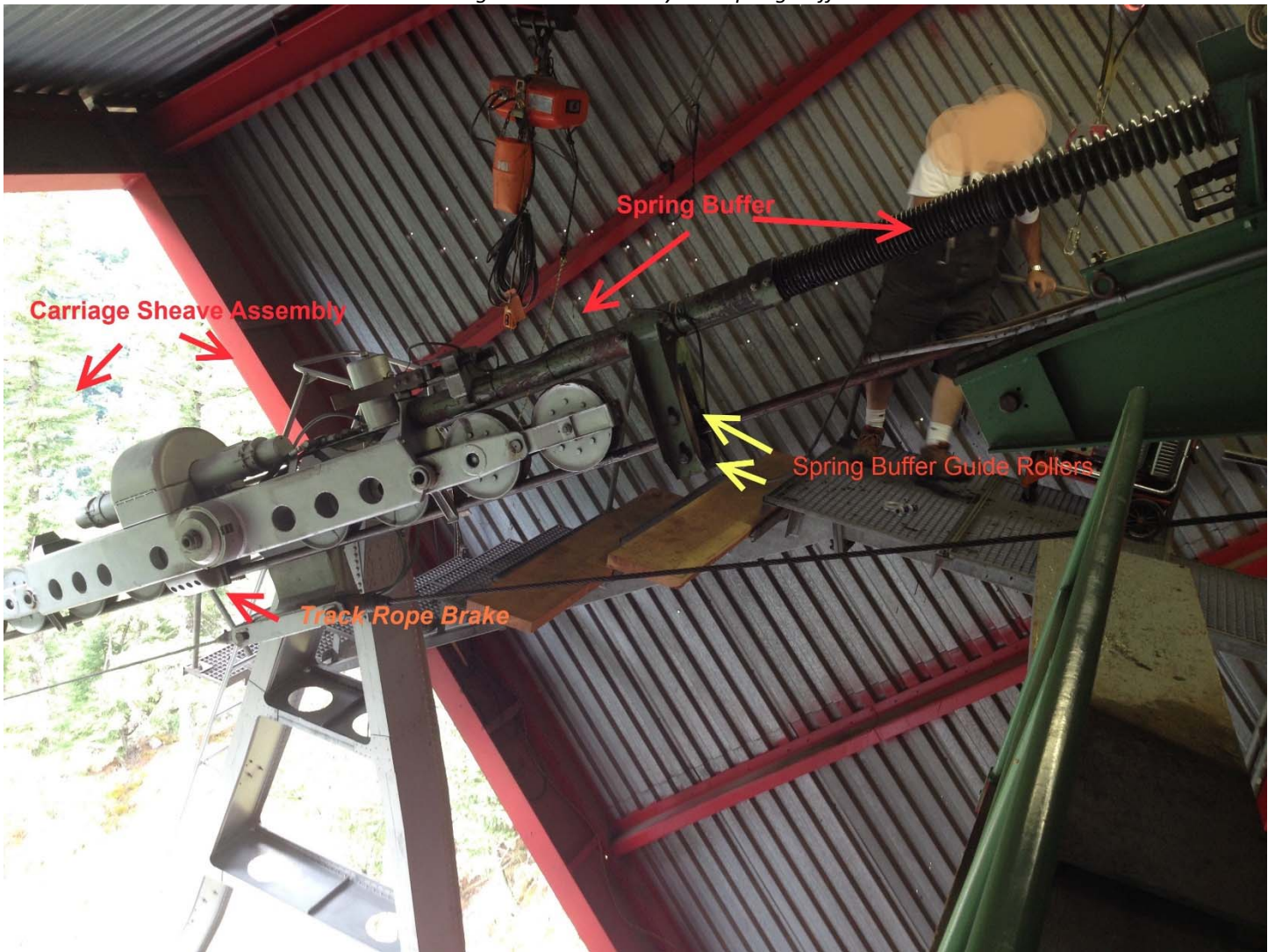
Carriage Sheave Assembly and Spring Buffer
