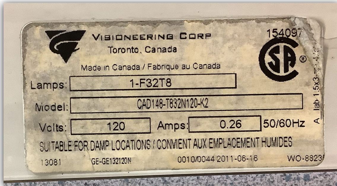
Image 1 - Label on the lighting fixture.
