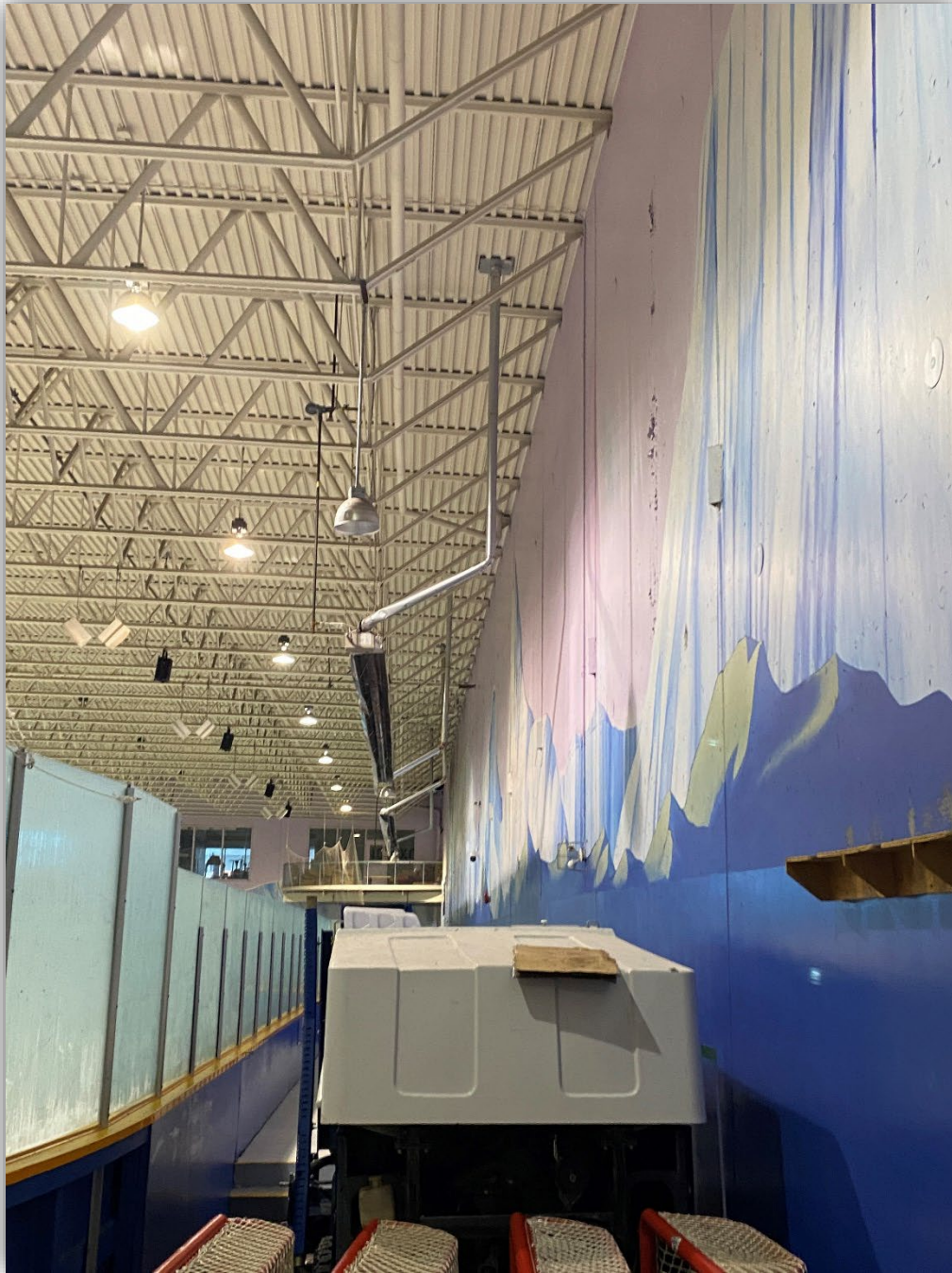
Image 2 – Two tube heaters above the spectator stands at rink 2.
