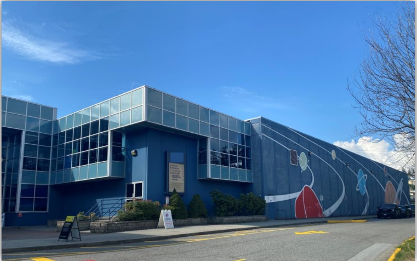
Image 1 – Outside of ice rink facility. The larger windowless building on the right houses ice rinks 1-2.
