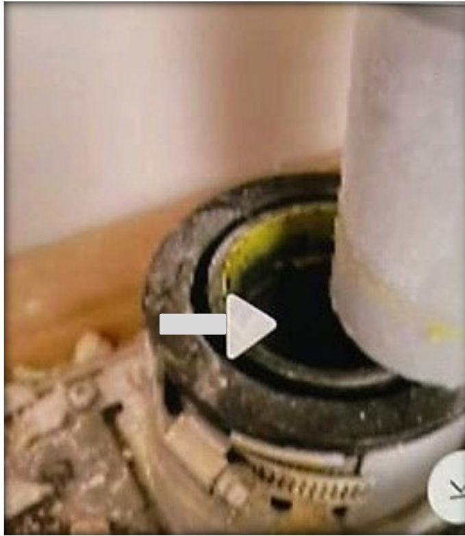
Image 6 - The PP vent dislodged from the black ABS reducing fitting on October 19, 2021.
