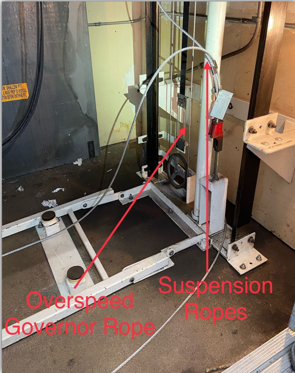
Image 2 - Overspeed governor rope & suspension rope.
