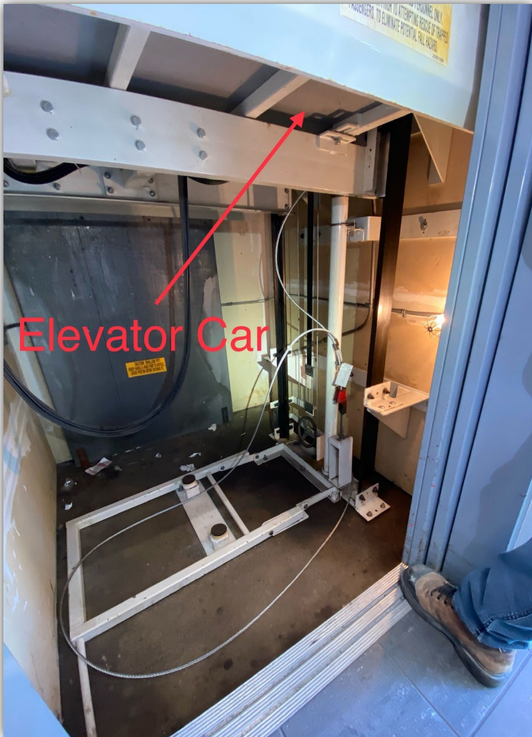
Image 1 - Elevator car from below.
