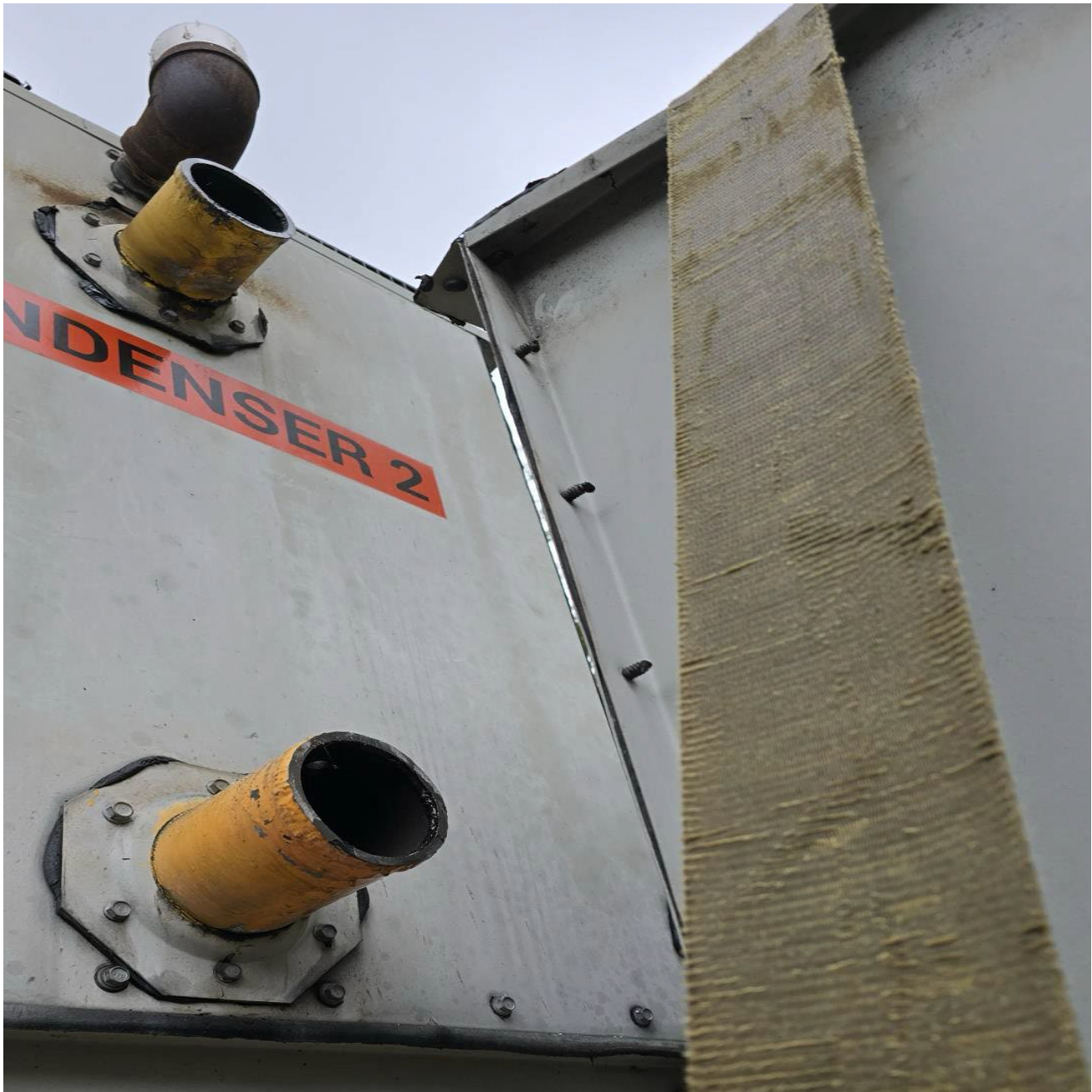
Image 2 - Condenser # 2 after removal from the structure.
