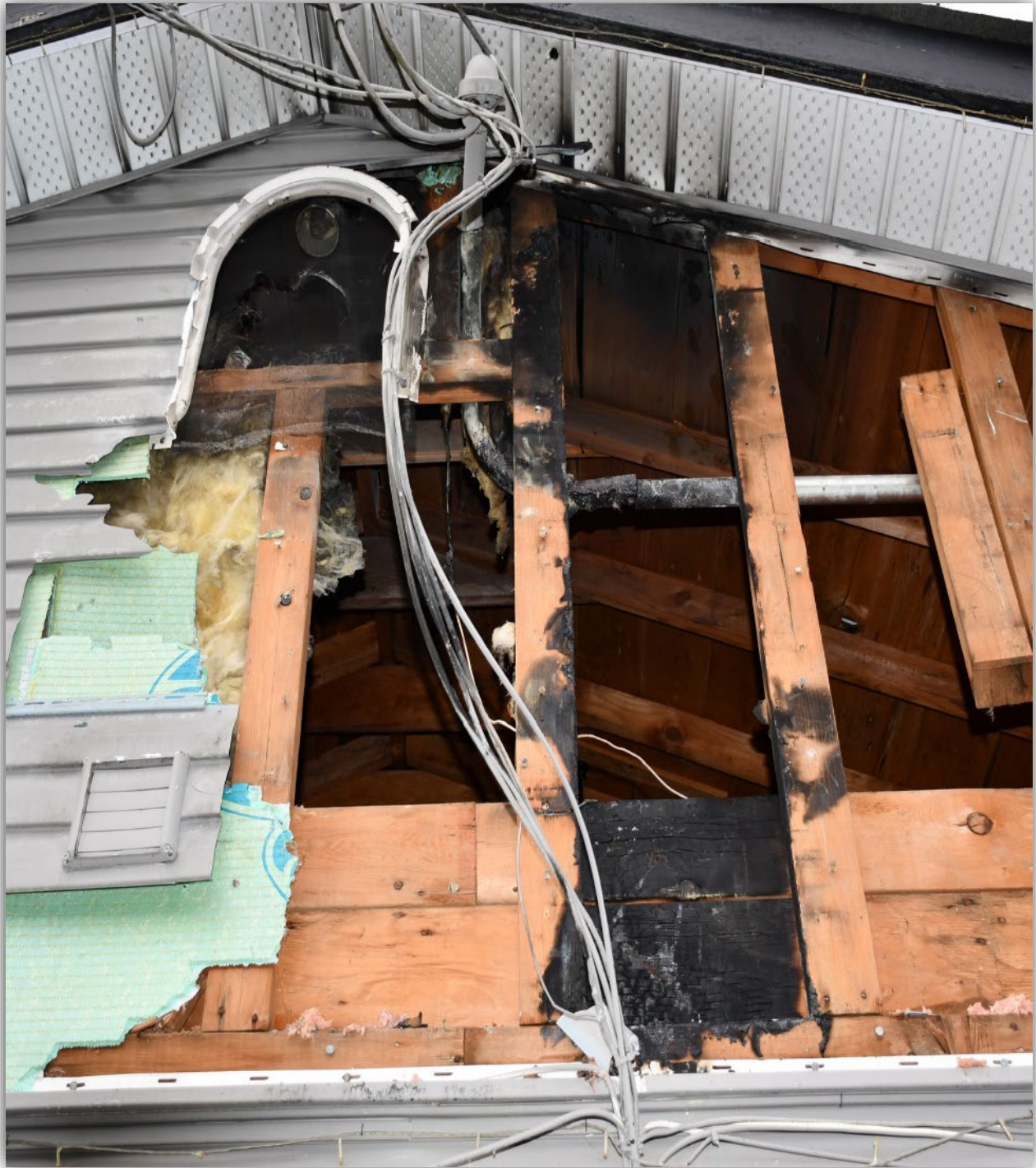
Image 2 - Fire started by molten drips. This is thought to be the area of origin.
