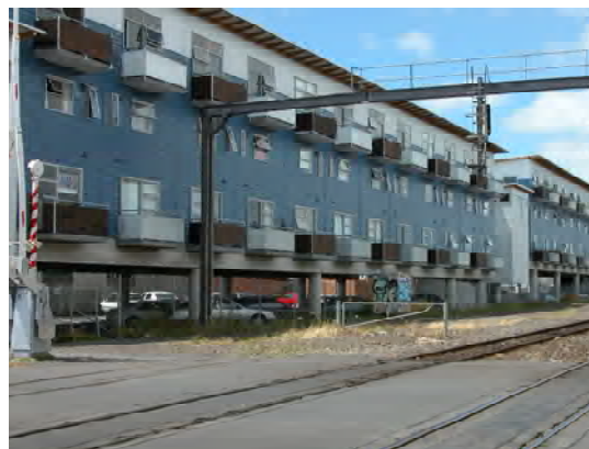
(iv) Medium-density housing along railway tracks, New Zealand
