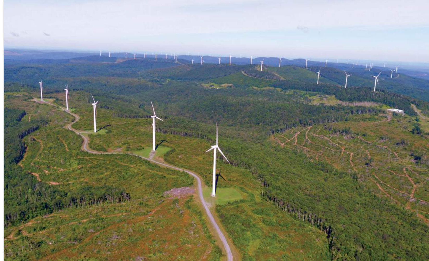
Beech Ridge II Energy Center (56.2 MW, Wind, WV)
