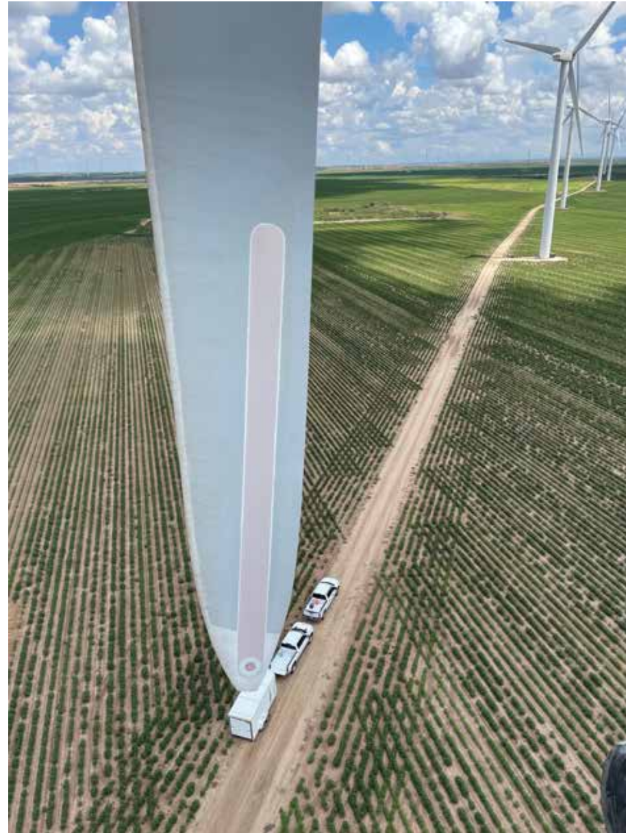
Lightening Protection System assistive tape adhered to one of our turbines.
