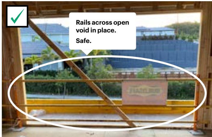
Timber/rails across void installed
