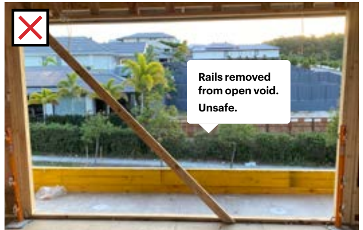
No timber/rails across void
