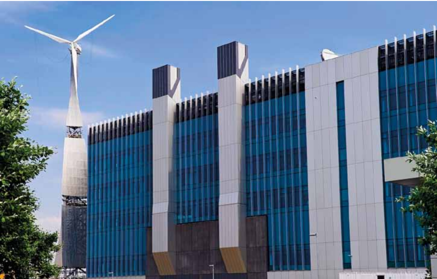
Sky Studios, Europe’s most sustainable broadcasting facility, opened in Summer 2011 at Sky’s London campus
