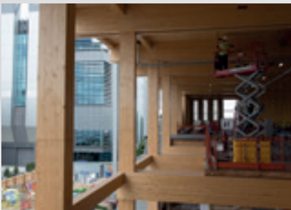
Sky Believe in Better building under construction
