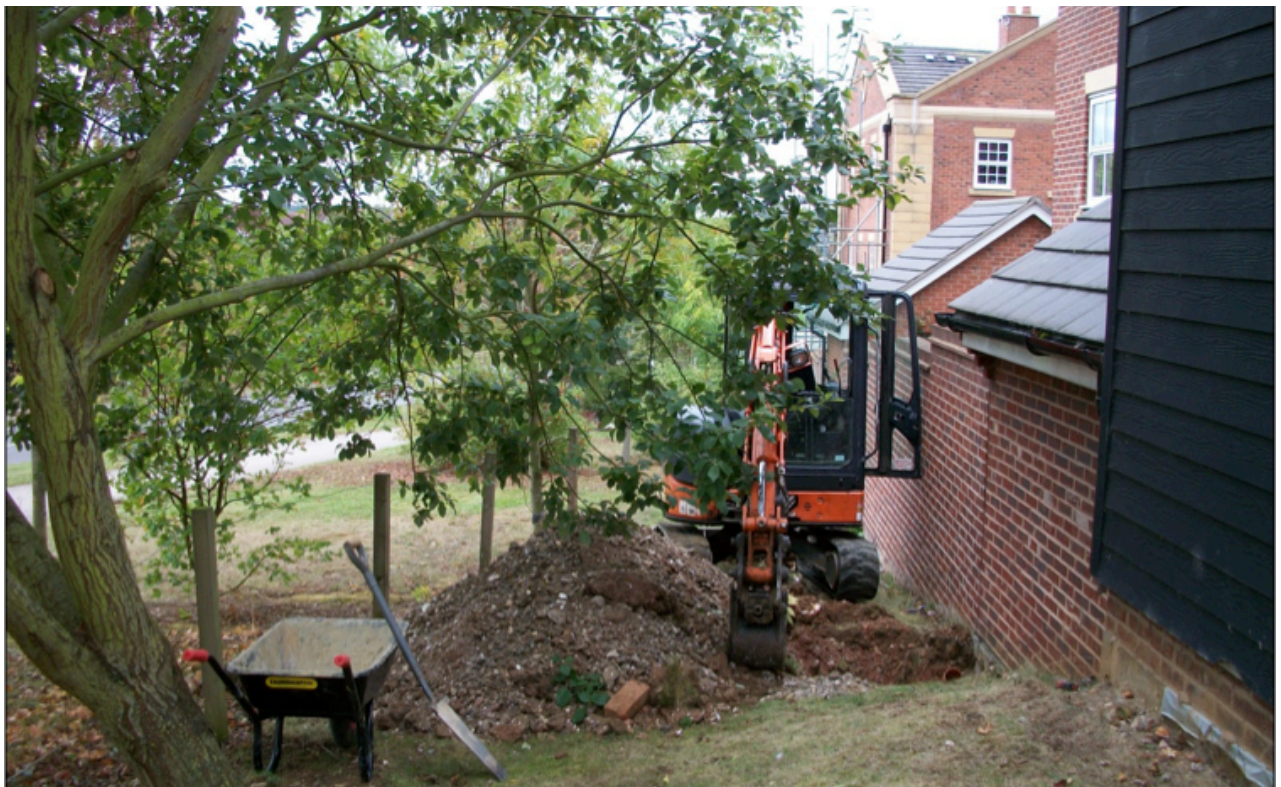
Intrusive investigations - Trial pits in progress to expose foundation formation level
