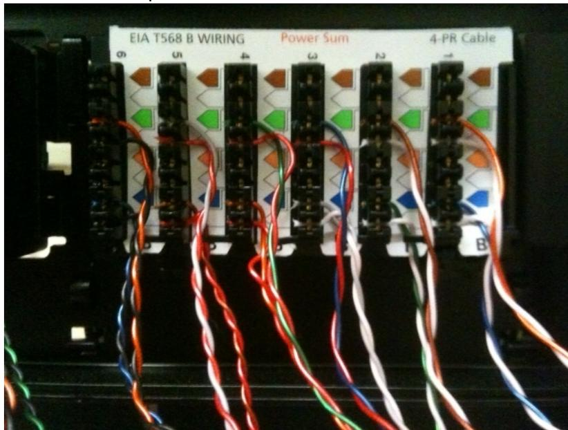
3. Feed panels will be labeled with a trunk identifier that matches the same feed location on the 110 punch field in the MDF.
