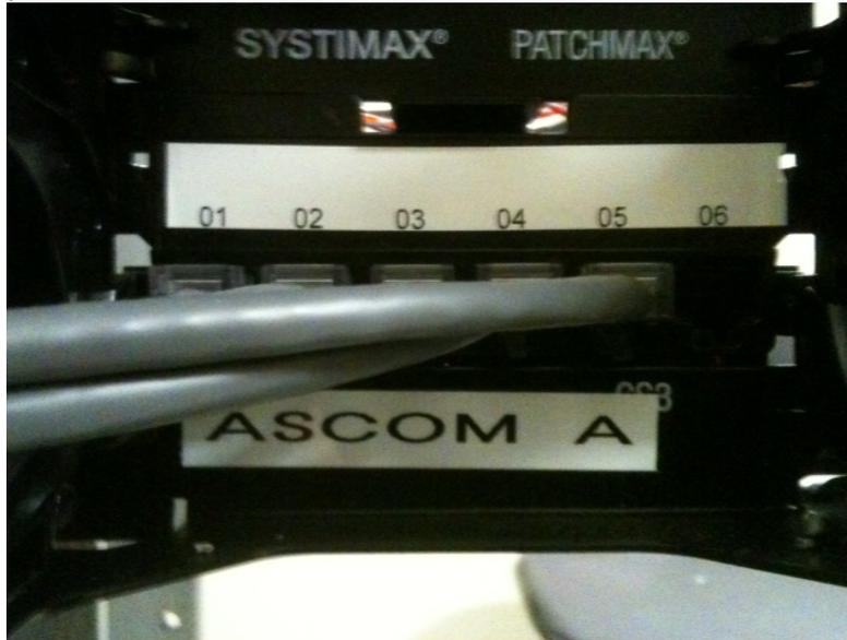
2. A dedicated 50 pair will be run to each closet from the PBX or MDF and terminated to its own patch panel with two pair per port, terminated on the Blue and Green pair.
