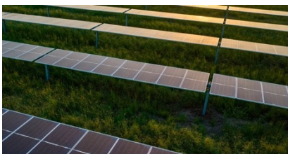
Invenergy's 100 th project, Southern Oak Solar Energy Center, located in Mitchell County, Georgia.
