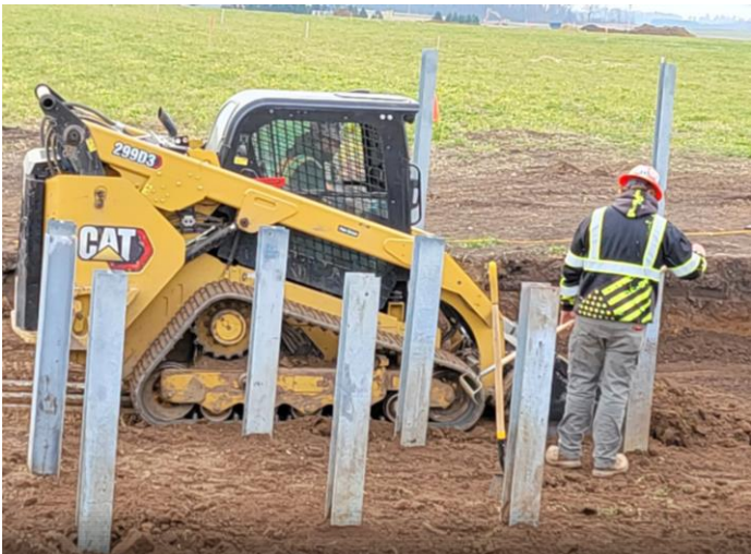
Construction of the inverter pad in the solar power block involves installing piles (shown) and a concrete pad to create a stable foundation for the equipment. Each of the 78 power blocks contains one inverter, which converts direct current generated by the solar panels into alternating current for the grid. Photo Nov. 24, 2025
