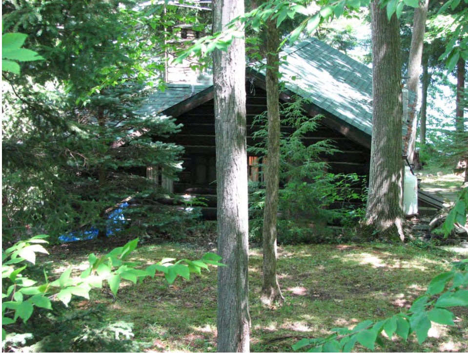
Photograph E.29. 8208 Lakeshore Drive ( Longiaru et al. 2007a ).
