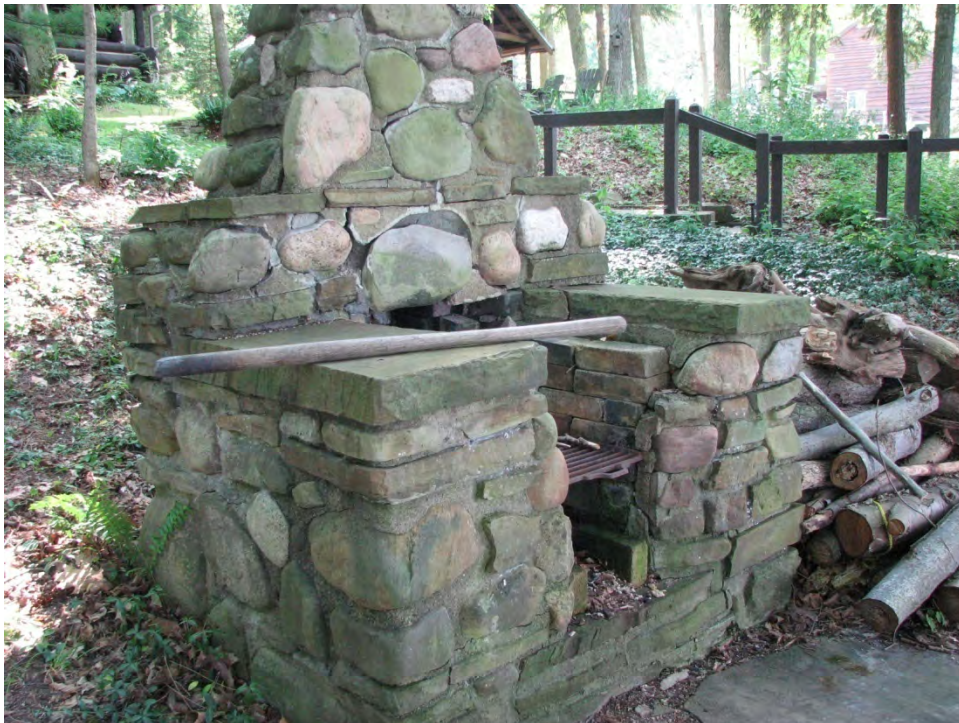
Photograph E.19. Exterior fireplace at 8204 Lakeshore Drive (Longiaru et al. 2007a).
