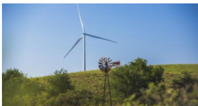
Invenergy-developed Conrail Wind Energy Center, located in Taylor and Page Counties, Iowa.
