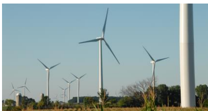
Invenergy’s Forward Wind Energy Center, located in Dodge and Fond du Lac Counties, Wisconsin.
